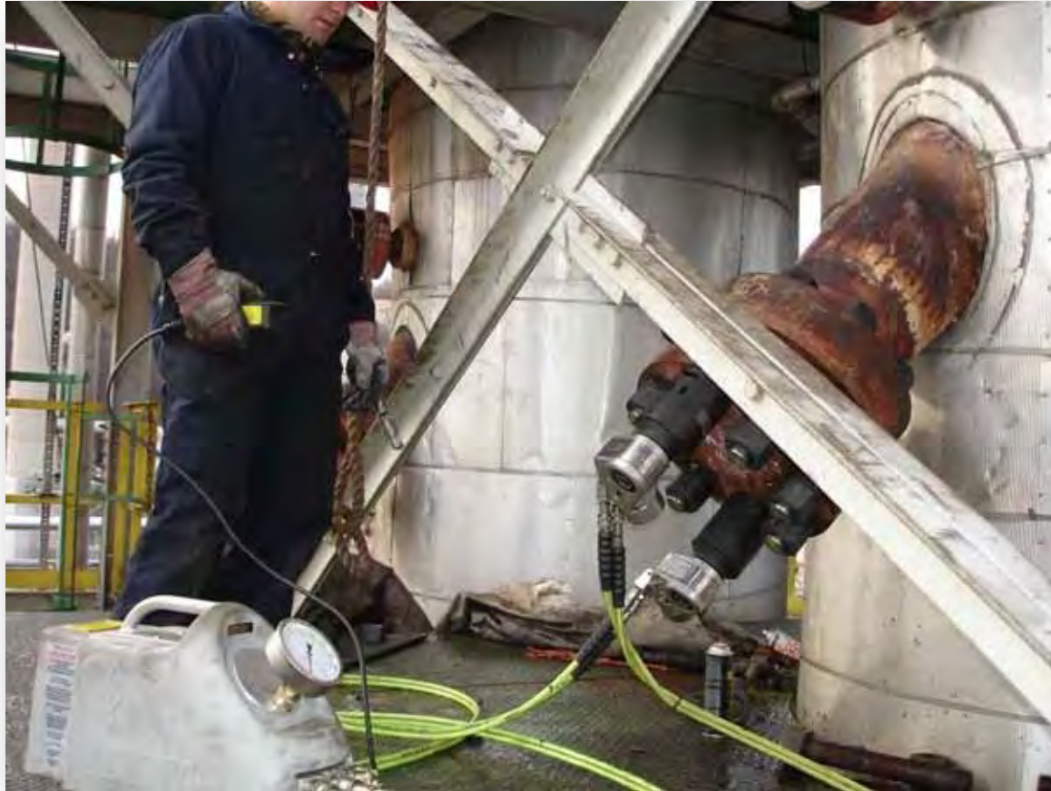
DUMP NOZZLE Bolting Made Simple
