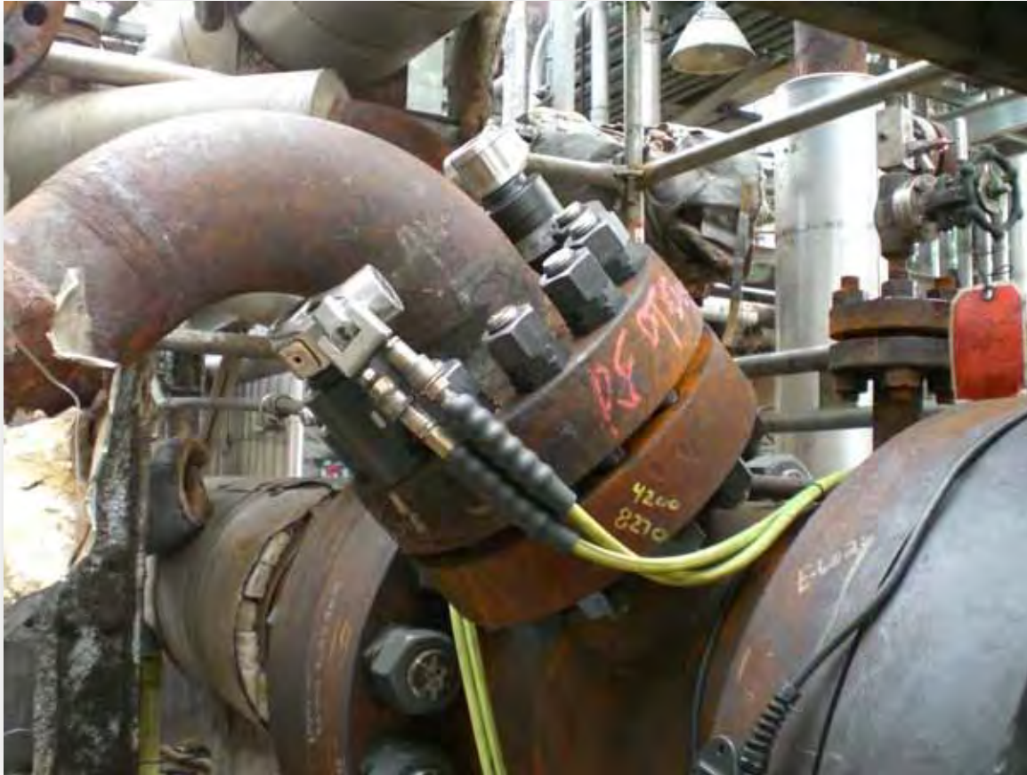
SHELL INLET-Via Remote Control
