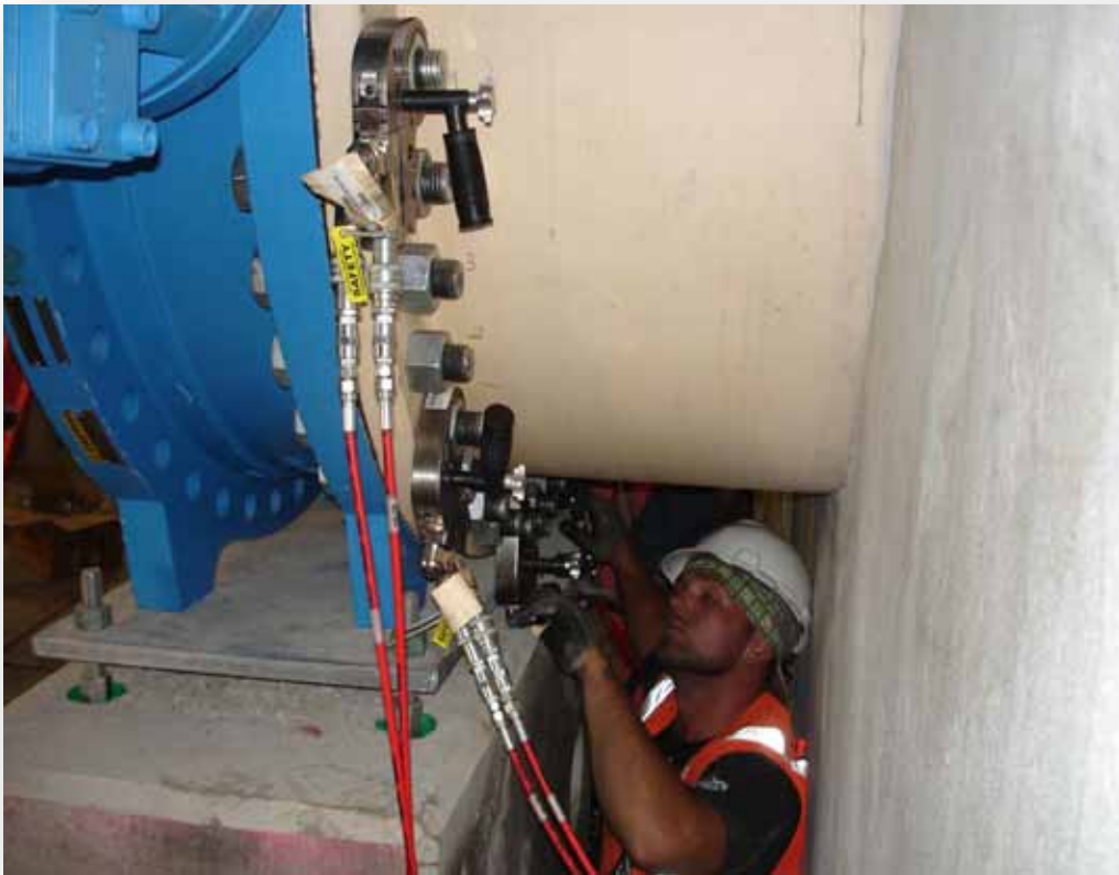
84" JOINT-Loaded with 11 Tool System
