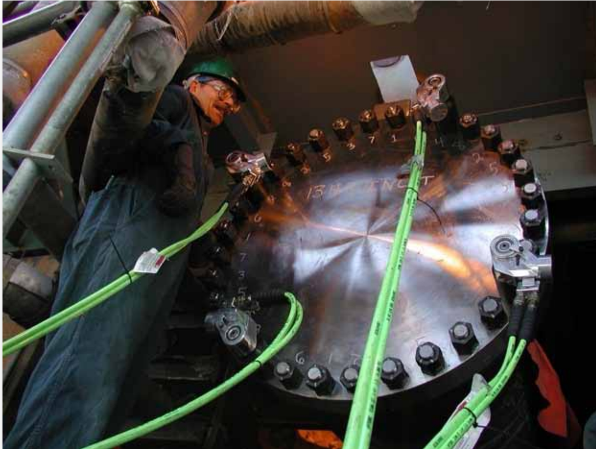
INLET HEADERS: Installed with HYTORC Precision
